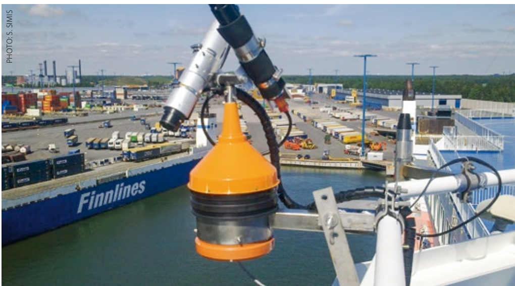
Installation of the Rflx system to collect data, BONUS FERRYSCOPE.
